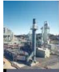
Kalina Waste Heat Plant
