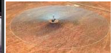
Concentrated Solar Power
