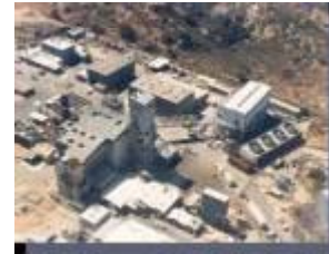
SCTI: Test Facility & Cogeneration Plant
